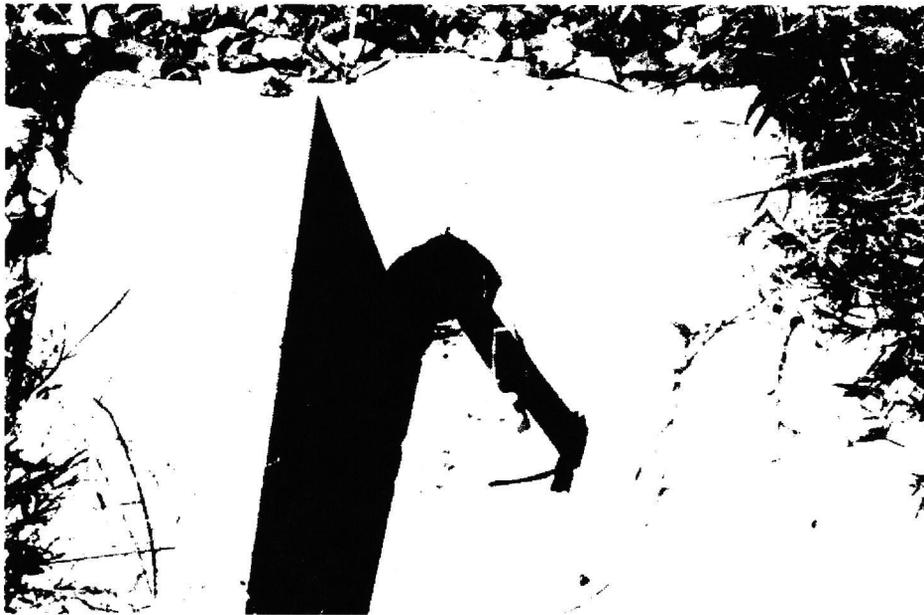
Picture 19. Edge Drain Outlet Pipe Damaged and Full of Material
